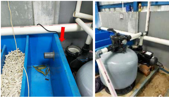
Fig 19: Position of the inlet pipe from the fifth shelter, connection from the pump to the sand filter. A: Water inlet from biological filter to water pump, B: Water pump to sand filter, C: Clean water from sand filter to water storage, D: Back wash or disposal water from sand filter
