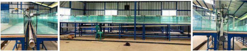
Fig 16: Installation of collector pipes for collecting wastewater from all aquariums
