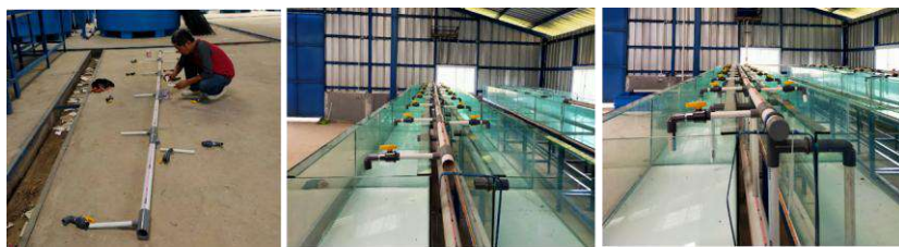
Fig 15: Installation of aquarium inlet pipes
