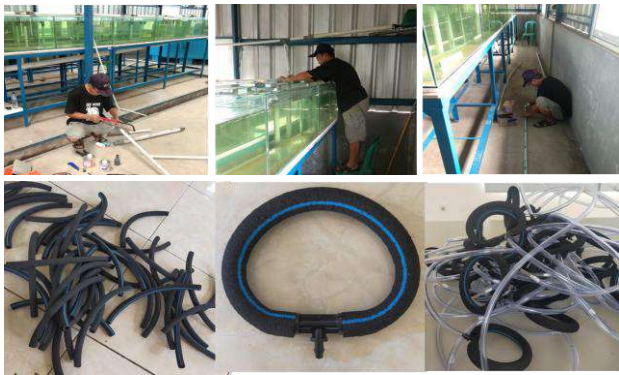
Fig 23: Installation of air distribution pipes from hi-blow, faucet installation and fabrication of "uniring bubble" air diffuser
