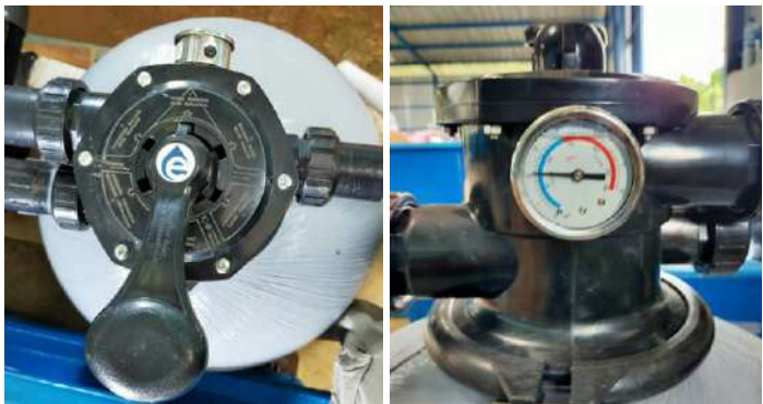
Fig. 20: Sand filter V200, mountain valve, amperemeter and connector pipes
