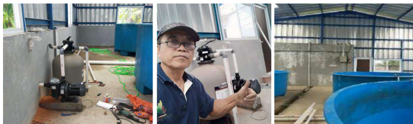
Fig 29: Installation of pump and sand filter in the broodstock rearing unit (left and center) and inlet pipe distribution to each tank (right)
